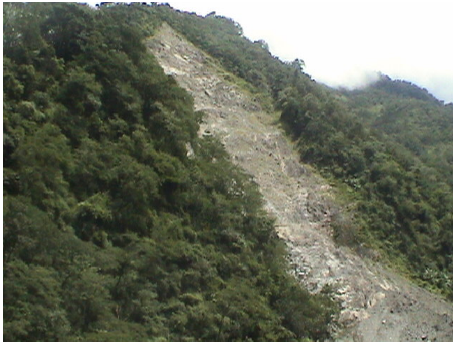
Photo 3.2: Active landslide zone near Airi Pani confluence with Dibang river (about 2 km u/s of Dam axis)
